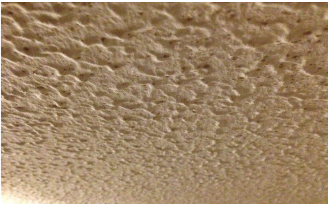
Sprayed asbestos on the ceiling of a school corridor – sprayed asbestos above suspended ceiling
