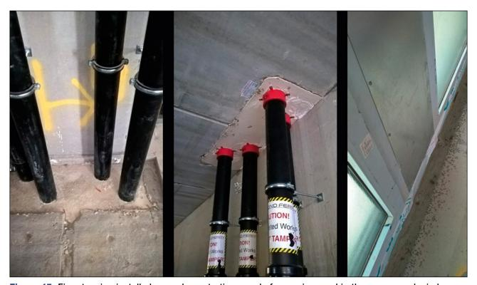
Figure 15 Fire stopping installed around penetrations made for services and in the gap around windows
