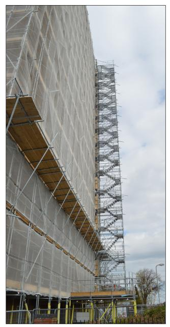
Figure 7 Where sheeted scaffolds form part of the escape route, do not sheet the stairways or ladder points so that smoke can escape and the fire and rescue service can gain access
