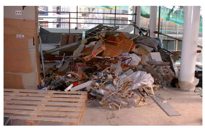
Figure 8 Most construction rubbish can burn. Make sure that it is cleared up and removed from the site as soon as possible
