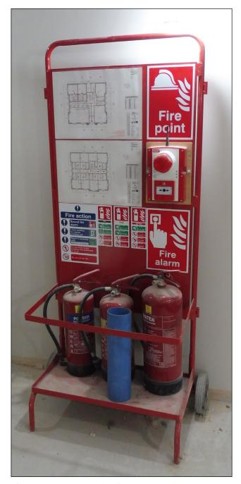
Figure 16 An example of an interconnected alarm and fire extinguisher point in a refurbishment project. Most sites will require an interconnected alarm system (either wired or wireless)
