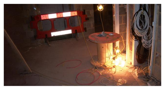
Figure 4 Festoon lighting: poor positioning creates a potential fire risk
